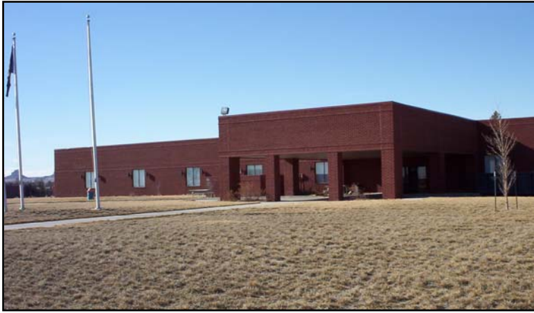
Future Home of Western Nebraska Community College's Center for Business and Individual Training
